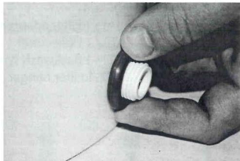
Place the o-ring onto the male threads on the outside of the bucket and screw the female adapter back onto the male threads.
