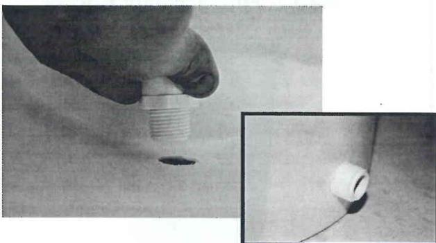
Place the male adapter through the hole inside the bucket so the threads are protruding to the outside of the bucket.
